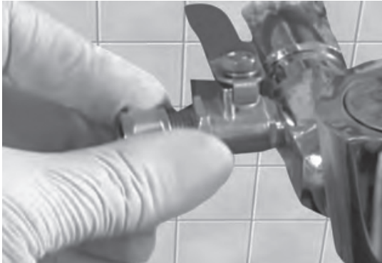
Figure 3.7 : Fixing valve in to 3 way connector
