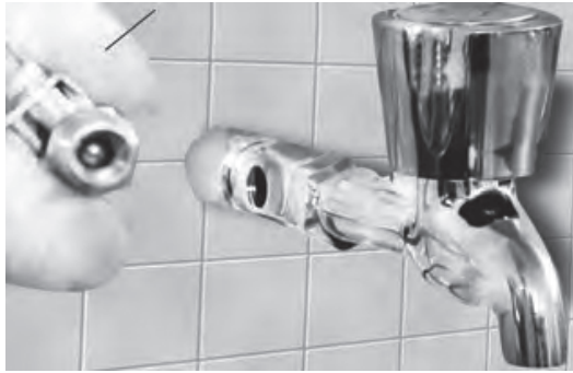
Figure 3.5 : Three way connection of water purifier
