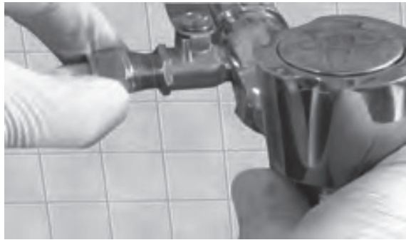
Figure 3.9 : Off position of supply line lever
