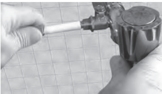
Figure 3.8 : Fixing tube in to outlet of valve
