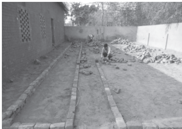
Fig. 3.7: Preparation of Loose Brick Vermibed
