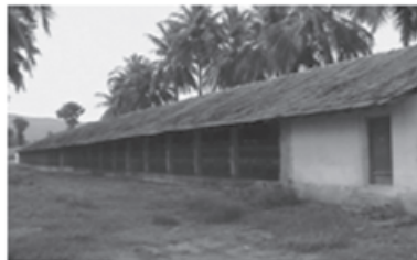
Initial tile roofed deep litter system house
