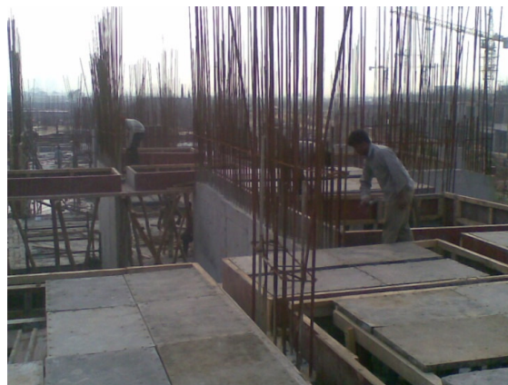
Fig. 11.4: Horizontal shuttering
