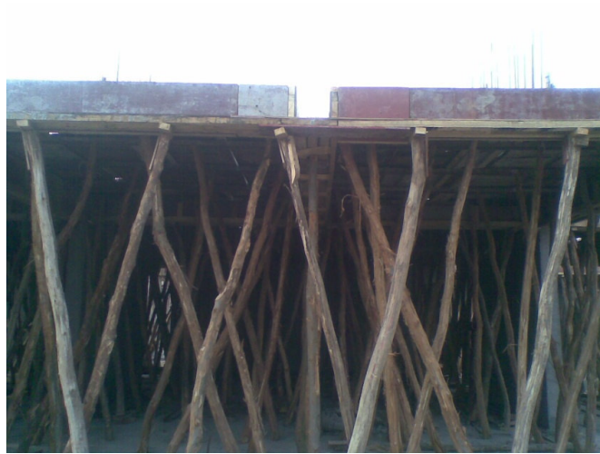
Fig. 11.3: Ballies below wood planks
