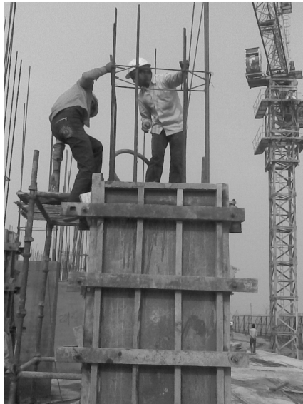
Fig. 11.2: Form work for column
