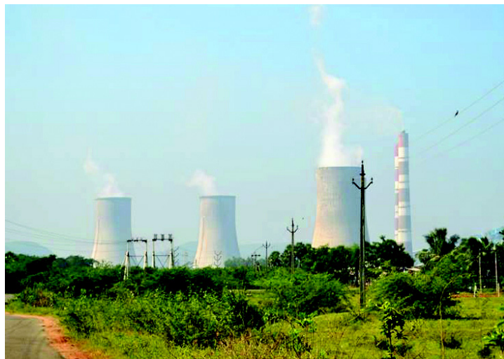
Fig. 9.6 Thermal Power Plant
